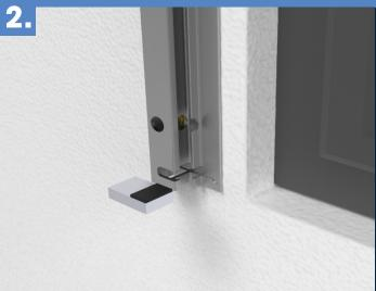
Stick the rubber strip to the support block as shown, before sliding the support block into position. Ensure the support block is sat correctly. The glass will rest on these blocks.
