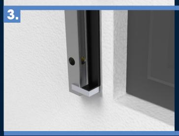
Remove the double sided tape paper from the foam strip and stick into the channel. This should be positioned directly above the support block for the entire length of the channel.
